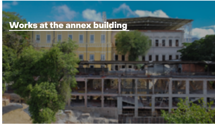
Progress in the restoration of the Paço
